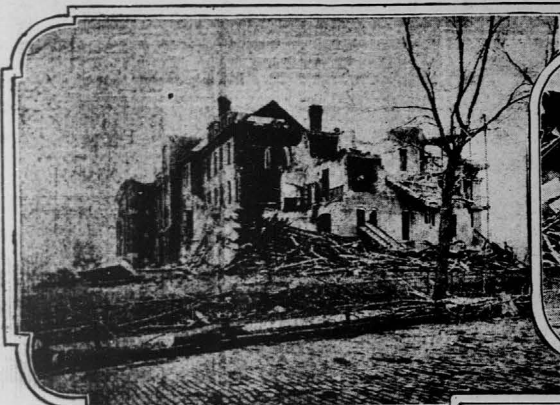
SACRED HEART CONVENT IN THE CENTRE OF THE FASHIONABLE CATHOLIC SECTION OF OMAHA, WRECKED BY THE TORNADO. PHOTOGRAPH FROM THE HERALD'S SPECIAL CORRESPONDENT
