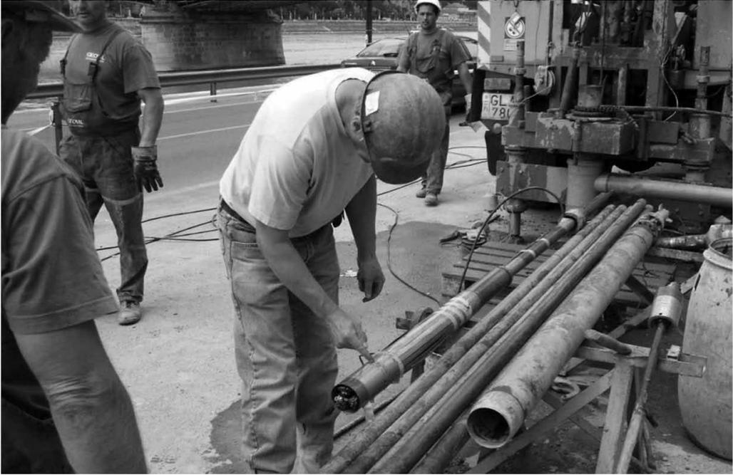
**Figure 5.** Selfboring pressuremeter
