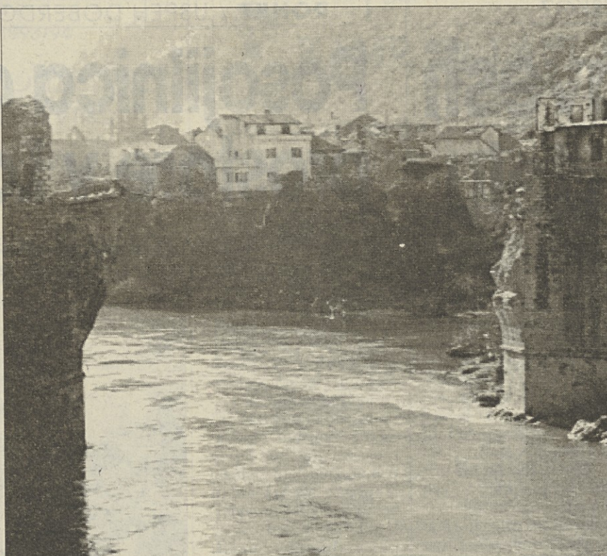
Porušeni most v Mostaru (Telefoto: AP)
