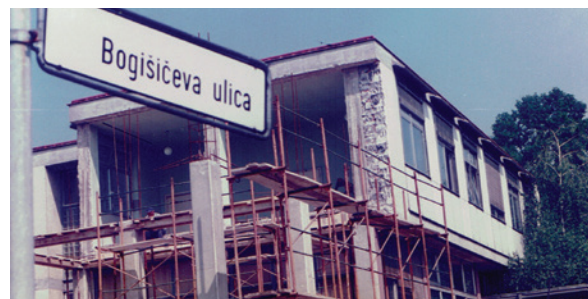
Gradnja ICP (inštitut za celulozo in papir) Construction of the ICP (Pulp and Paper Institute)
