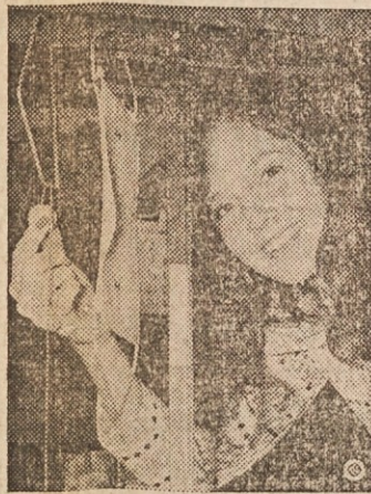
TESTING —Maid of Cotton Debra Ploch checks out the dimensional stability of a cotton knit fabric at the Southern Regional Research lab in New Orleans. The device she's operating measures the degree to which a fabric holds its original size and shape after being placed under tension for a prescribed length of time.
