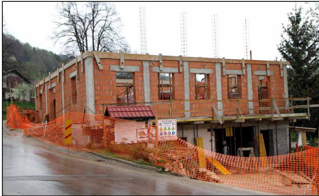
PGD Velika Pirešica gradi nov gasilski dom.
