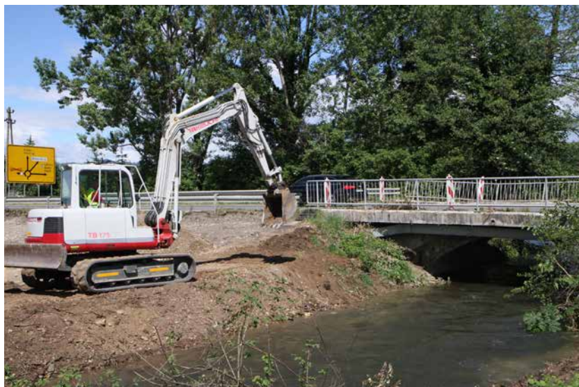
Dotrajan most čez Strugo bodo obnovili, pred tem pa zagotovili nadomestni most
