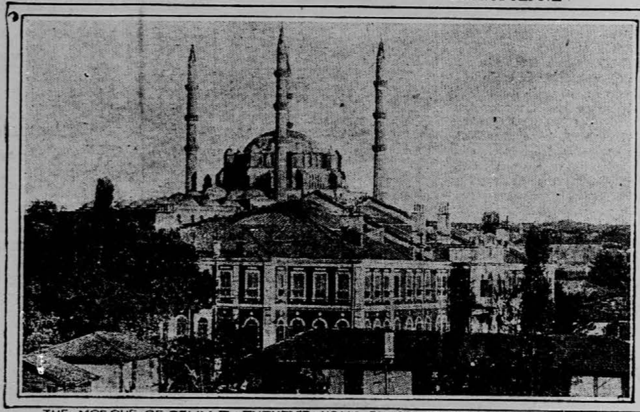
THE MOSQUE OF SELIM II. TURKEY'S HOLY PLACE AT ADRIANOPLE
