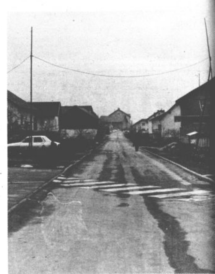
..... in asfaltirane ulice.
