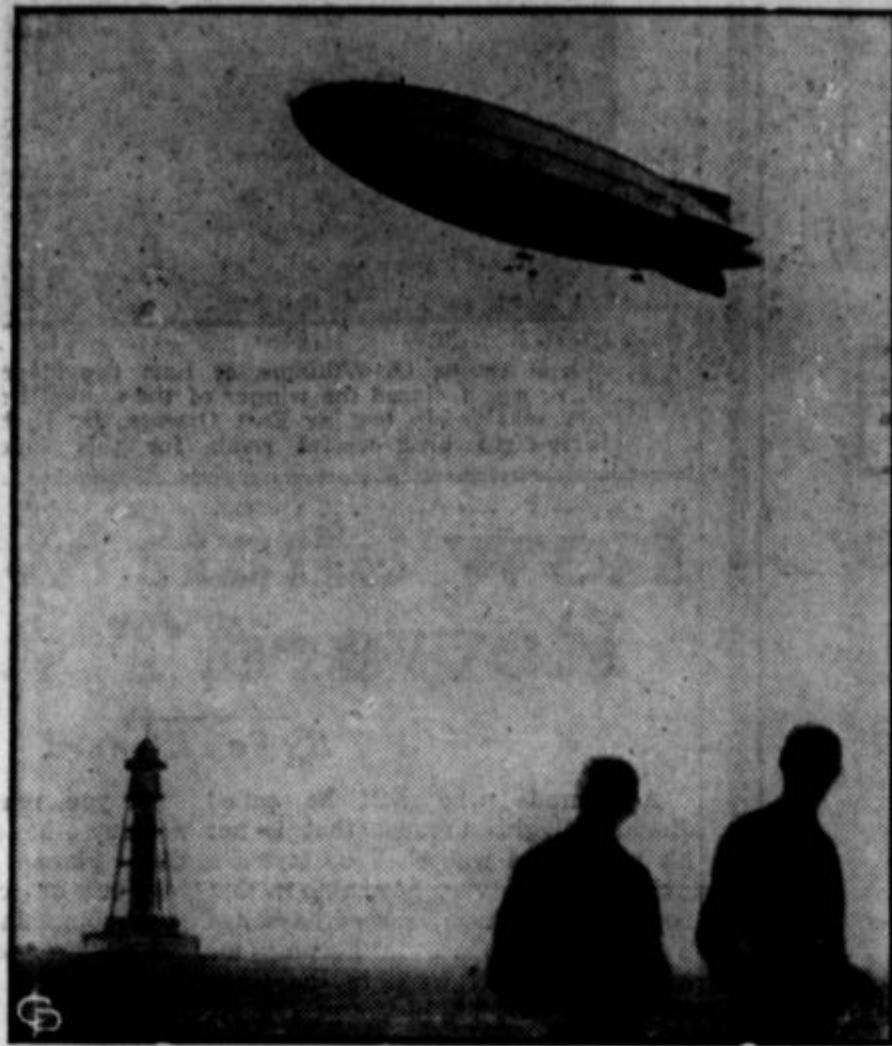
The storm-tossed R-100 photographed as it neared its Montreal mooring-spire after its epochal flight from Cardington, England. The big English ship, largest dirigible in the world made the trans-Atlantic voyage in 78 hours and 51 minutes. It reached the Canadian city with a broken tail fin.
