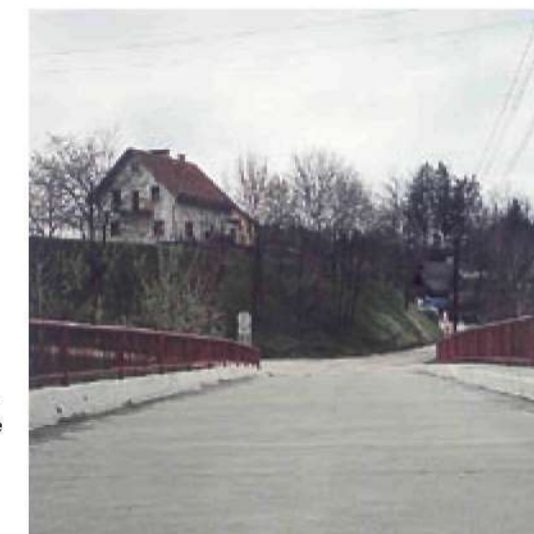
Figure 8: Overlay on the bridge over the Kokra River in Kranj.
