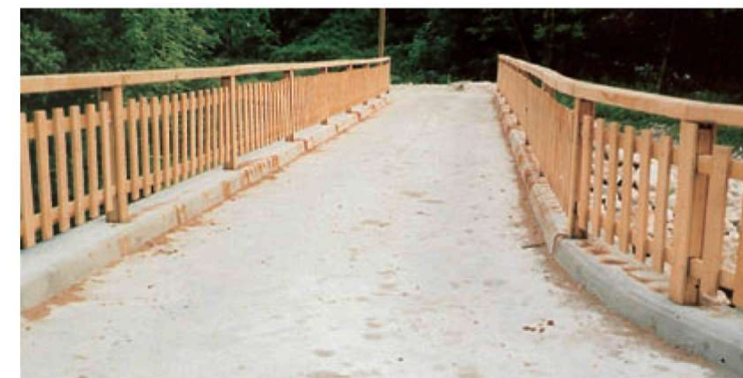
Figure 9: Overlay on the bridge over the Soča River near Podbreg.
