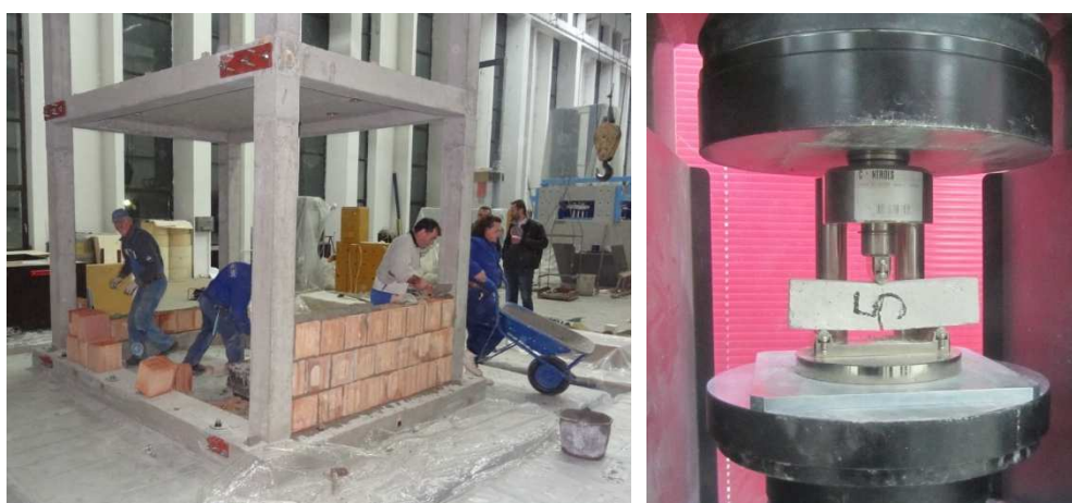
Slika 6.6: Izdelava opečnih polnil in test upogibne trdnosti malte Figure 6.6: Masonry infill construction and mortar bending strength testing
