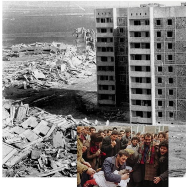
Figure 2.1: Large panel precast structure standing among the rubble of the precast frames that caused a tragedy during the Spitak 1988 earthquake (Fischinger et al., 2014)
