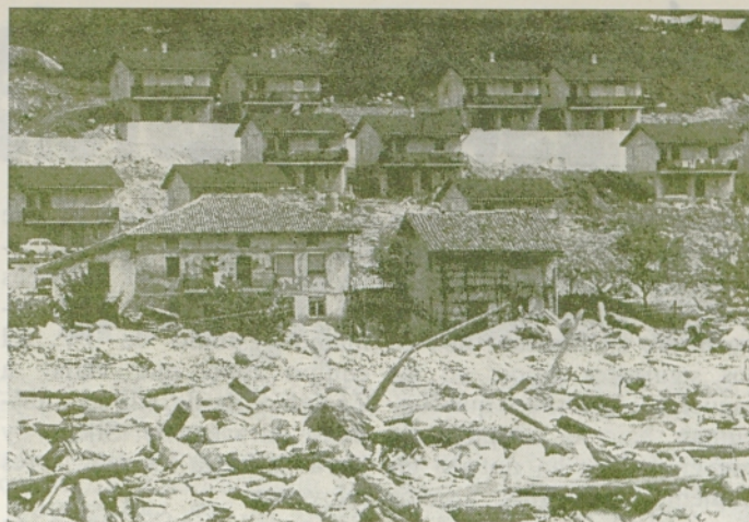
The village Breginj rebuilt after earthquake
