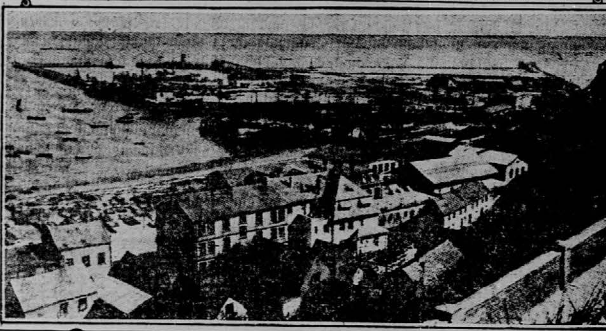
THE NEW HARBOR AT HELIGOLAND
